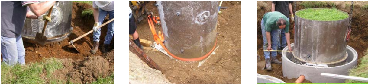
Figure 2. Control of cutting edge, shearing and excavated monolith
